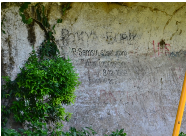
Figure 6. Vandalism observed in the wall of Gunung Reng hill.
